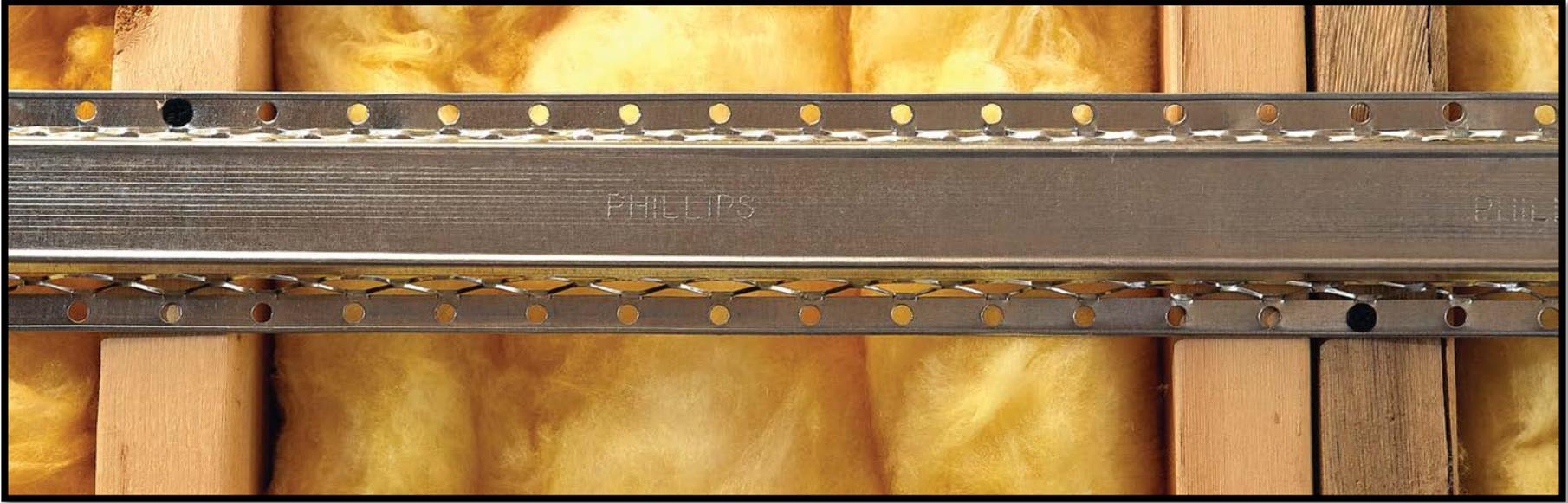
**Attachment flanges must remain face down**, ensuring the open side of the RC is face up towards to top of the wall.
